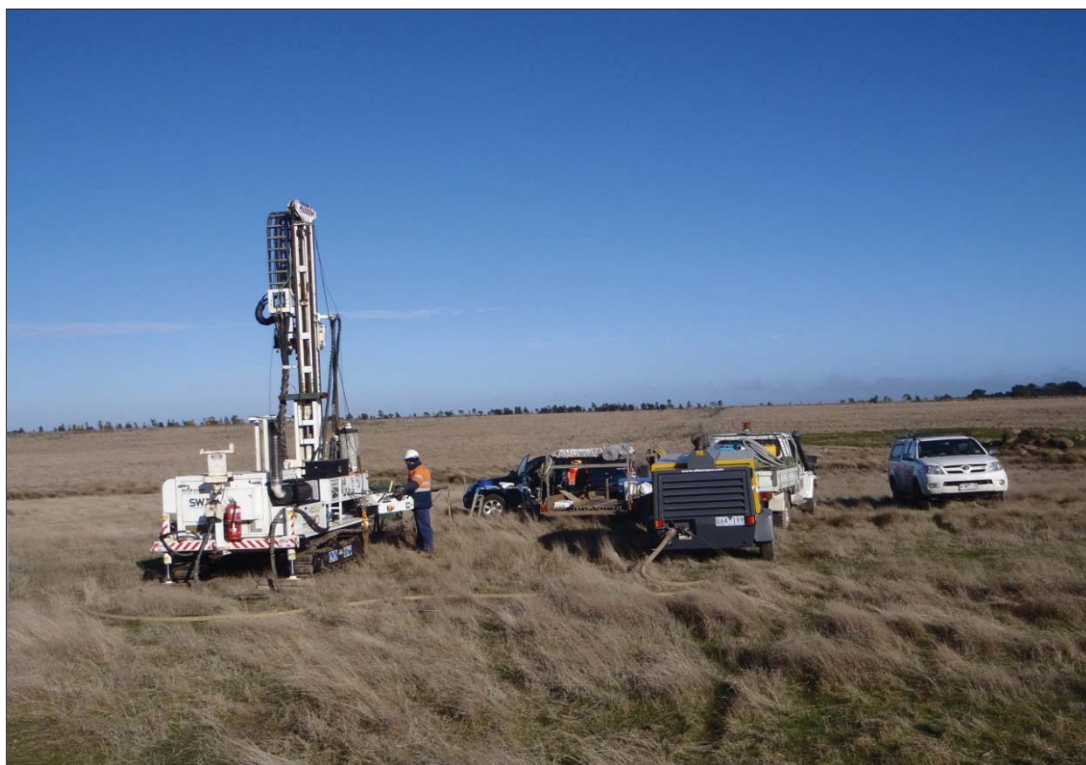
Figure 4-1: Drilling of Groundwater Bore GW102
