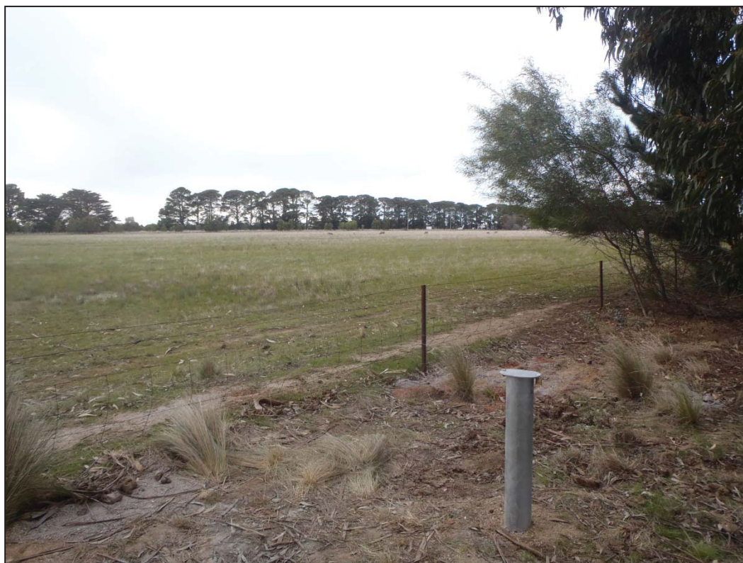
Figure 4-2: Protective Cover on Bore GW104
