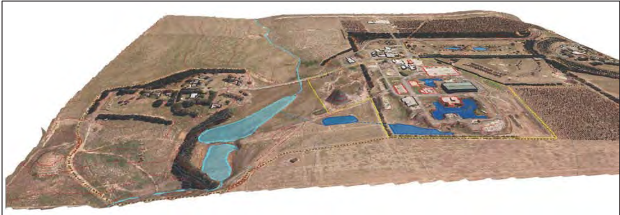
Figure 2-1: Oblique Aerial Photo of Site
