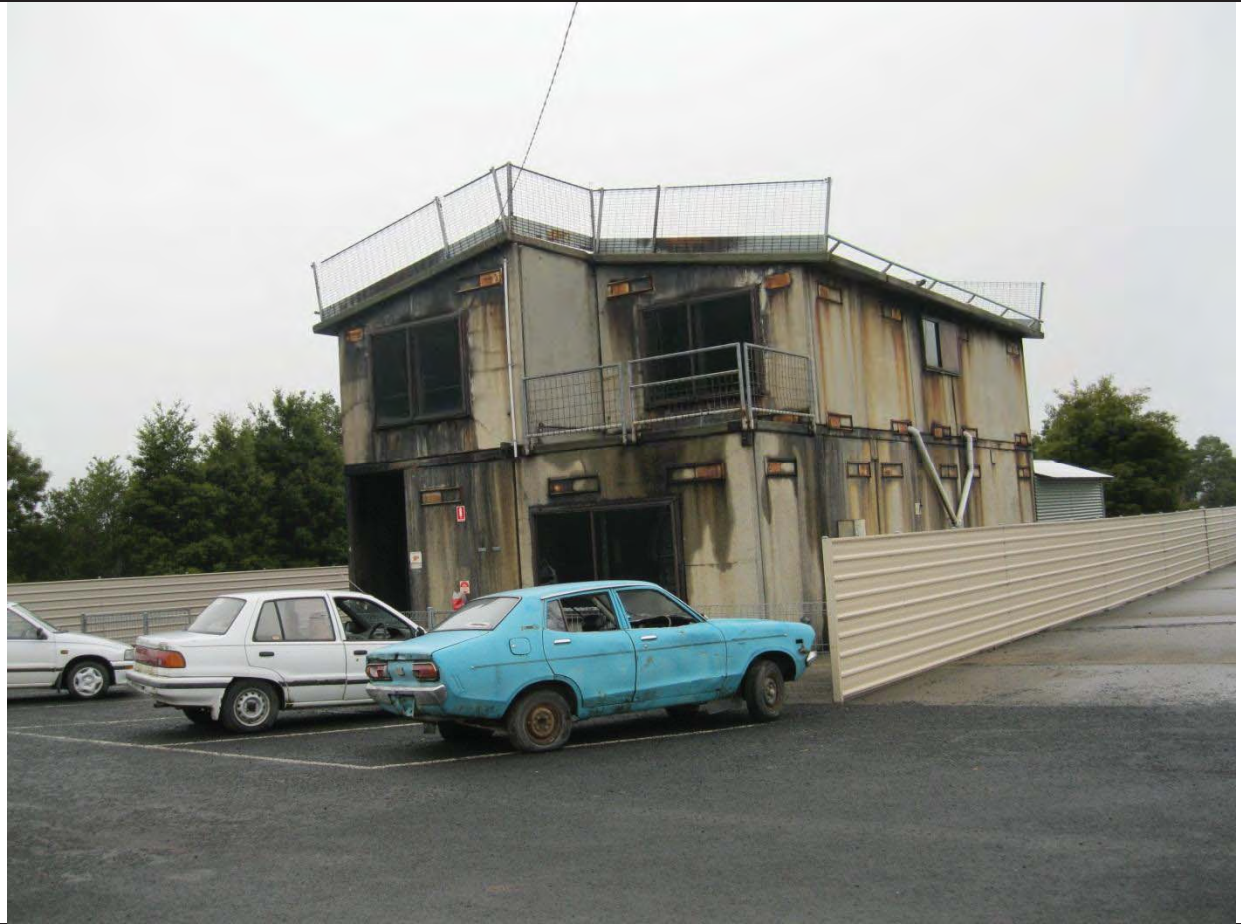
PLATE 9 Structural Fire Attack Building (Feature 33b) looking south-west
