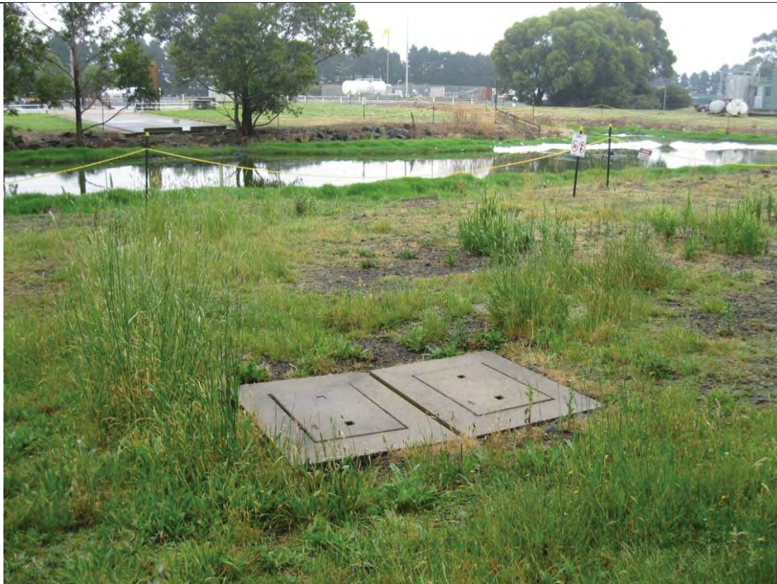
PLATE 6 Effluent pit inspection covers between Dam 1 and the VUT building
