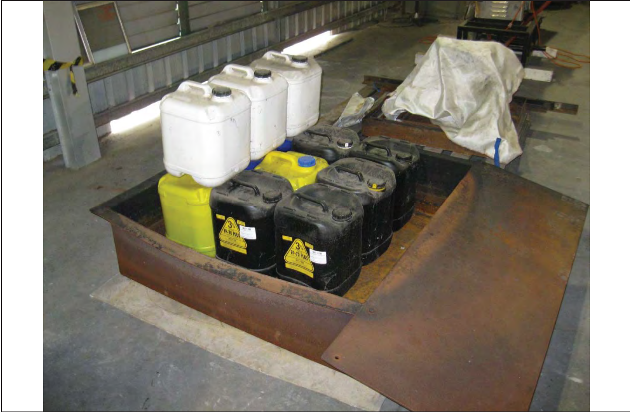
PLATE 7 Foam concentrate in bunded Storage area -
