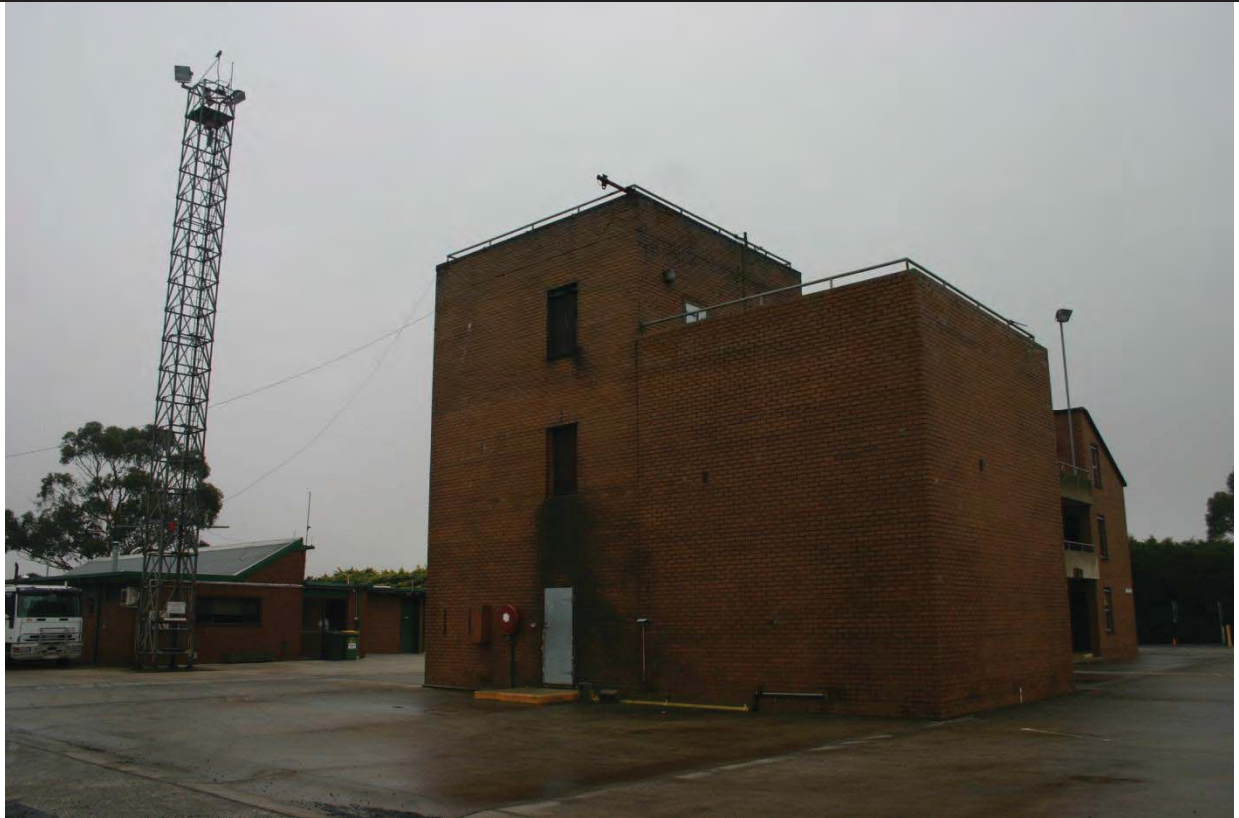
PLATE 8 Fire Attack Building (Feature 24) looking north-west
