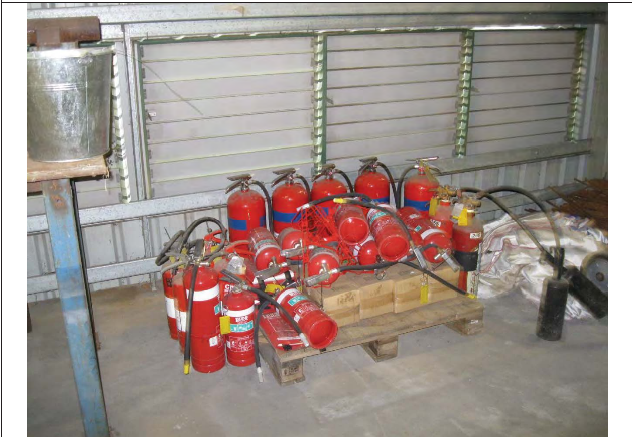
PLATE 8 Dry chemical fire extinguishers
