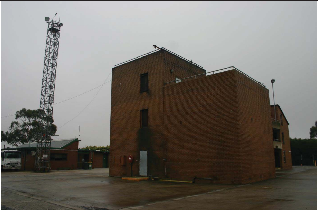
PLATE 10 Fire Attack Building (Feature 24) looking north-west
