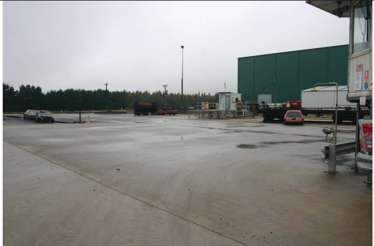
PLATE 5 Flammable Liquid PAD (Feature 27) looking south-east
