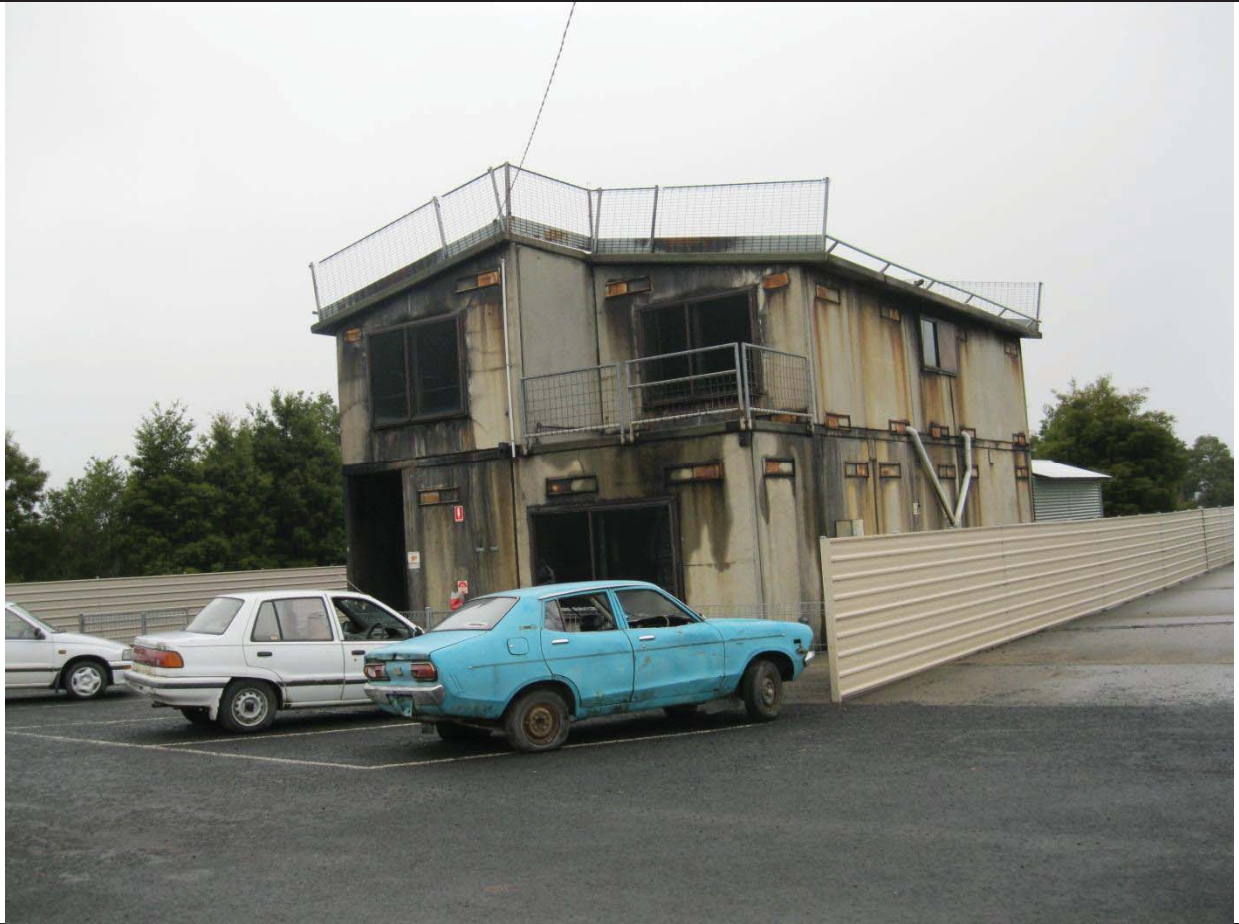
PLATE 11 Structural Fire Attack Building (Feature 33b) looking south-west
