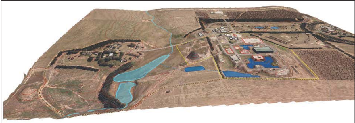
Figure 2-1: Oblique Aerial Photo of Site
