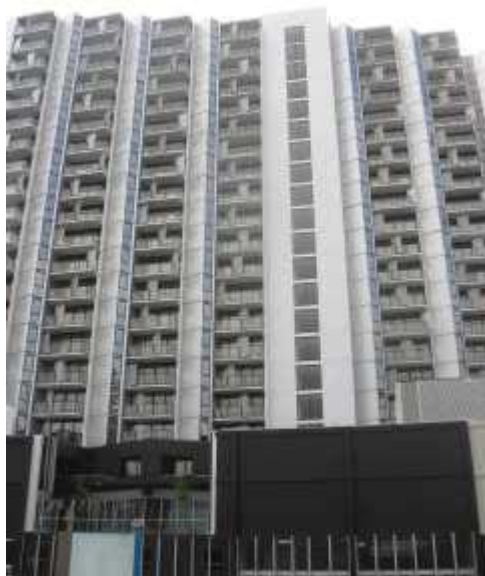
Photo Prior To Fire
