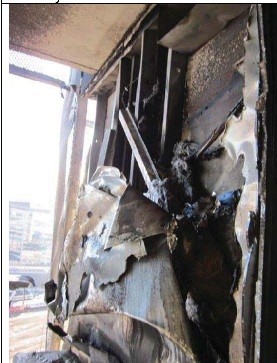
External wall at upper height
