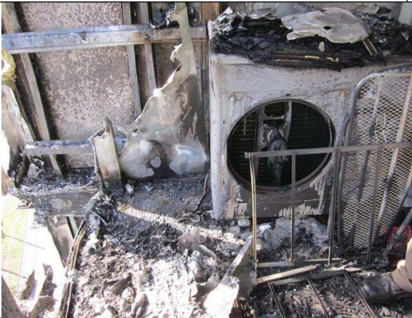
Photo of base of wall and penetrations plus overhang past balcony edge
