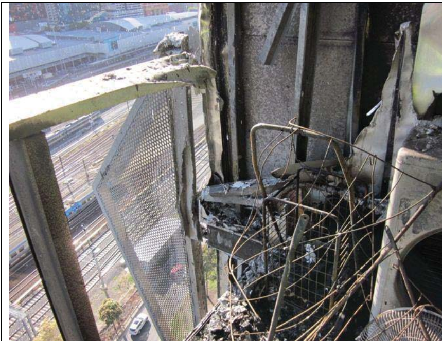
Wall between bedroom and balcony. Construction lightweight wall with steel studs, aluminium type external cladding plasterboard to internal. Material stored on balcony.
