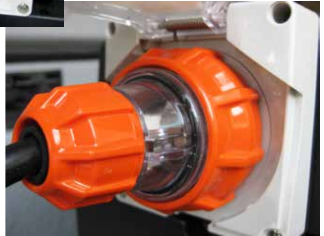
← An IP66 rated Mode 2 outlet (cover open) and ↓ threaded IP rated 3-pin plug inserted and screwed in.
