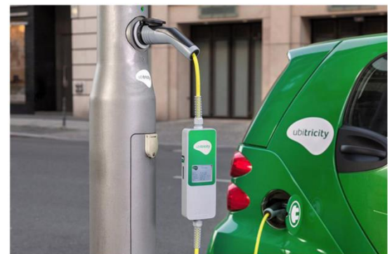
Figure 5: Ubitricity Street Light Charge Point (source: Web Urbanist 2017)
