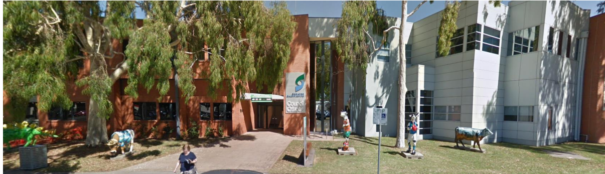
Figure 42: Greater Shepparton City Council Offices (source: Google Street View)
