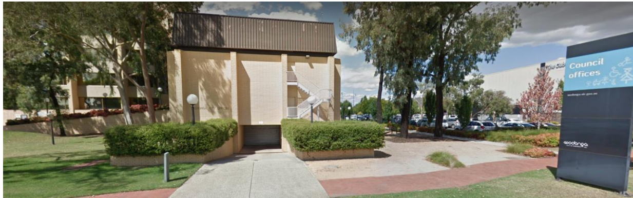
Figure 54: Wodonga City Council offices (Source: Google Maps)
