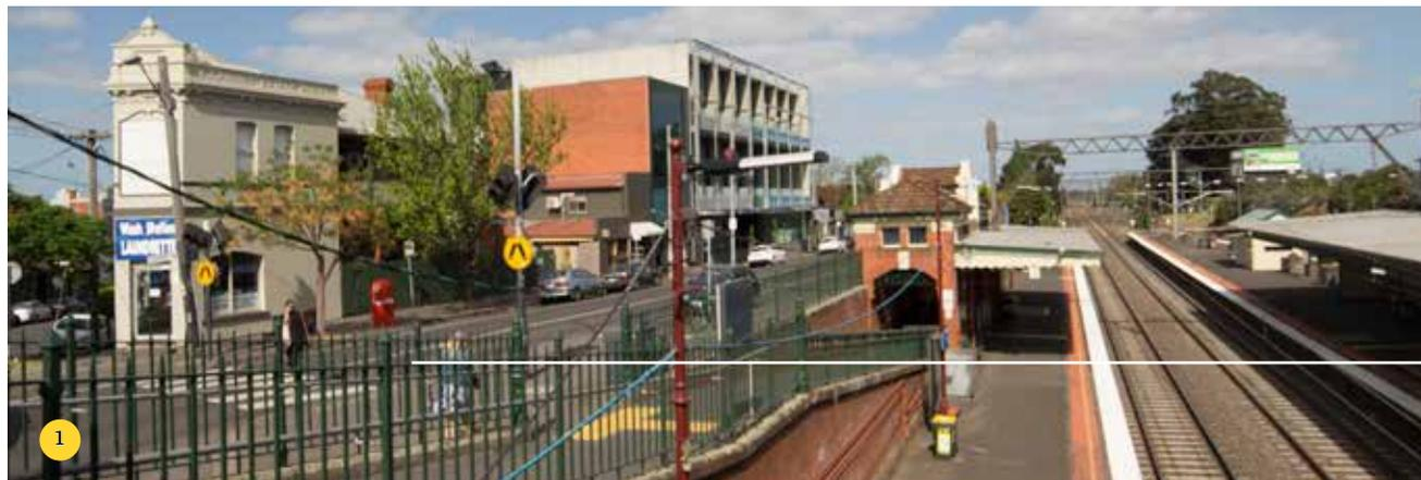
Malvern Station was re-built in 1902 as part of the major re-grading and track upgrade between South Yarra and Caulfield to improve rail capacity. Most of the corridor was placed in a wide trench. The streetscape is discontinuous across the railway trench and the station is poorly integrated with it nor easily accessible to its trams.
