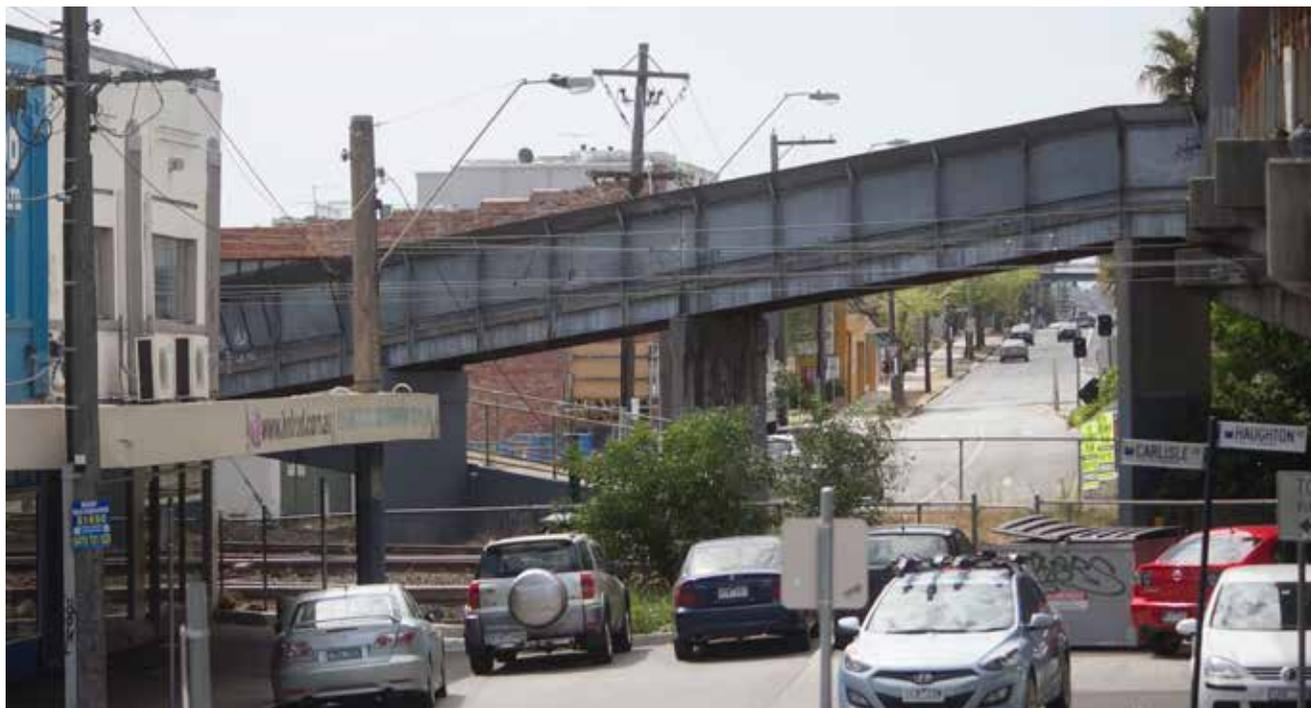
Pedestrian ramps, Oakleigh Station, due to discontinuance of ground level connectivity after level crossing removal (2015)
