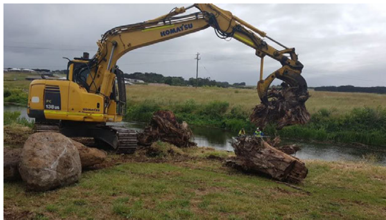
Root balls and rock piles being installed in the Merri River Estuary. Credit: S.Ryan
