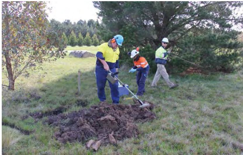
Figure 4-2: Metal Detector Scanning EM Anomaly during Intrusive Investigations
