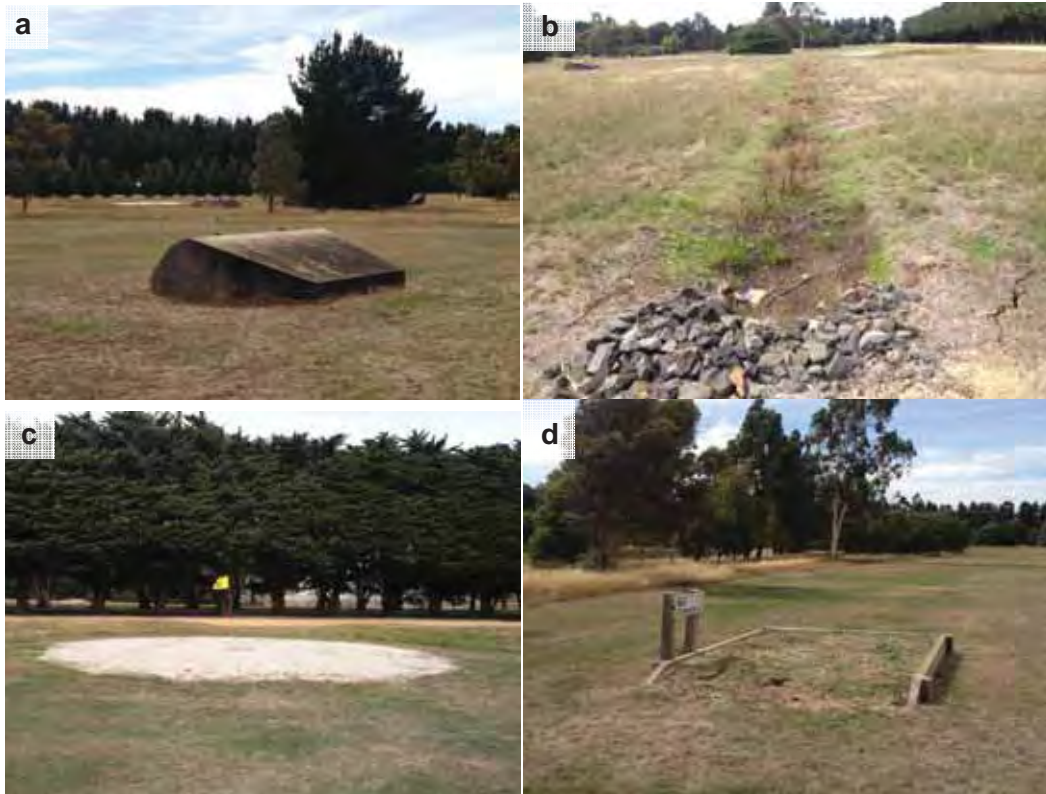
Figure 2. Major features of the Drum Burial Area 3a including: a) concrete cable anchor, b) drainage ditch, c) golf hole & surrounding mounds and d) raised golf tee.
