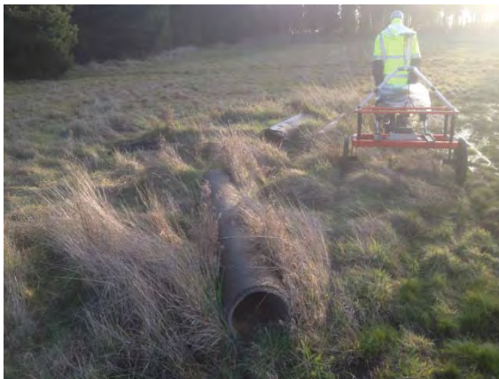
Figure 6. Reinforced concrete pipes located on site Drum_Burial_Area 1.
