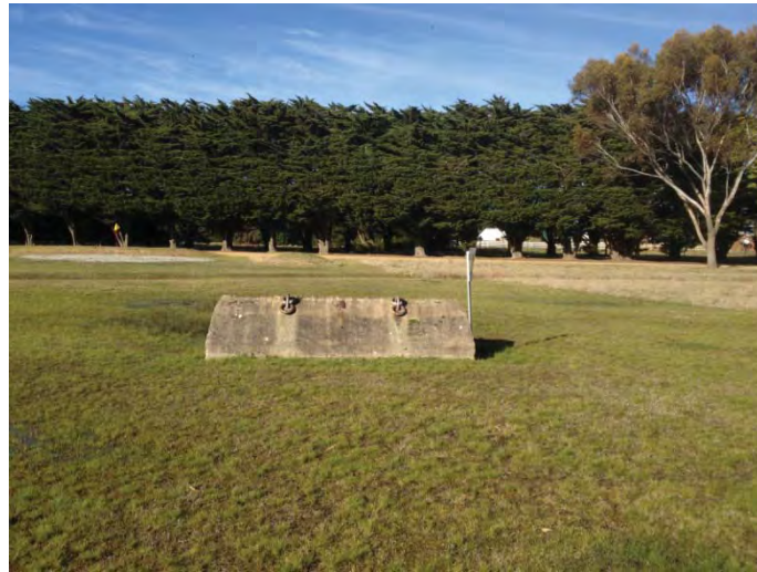
Figure 8. Former radio tower anchor located adjacent to site Drum_Burial_Area 3.
