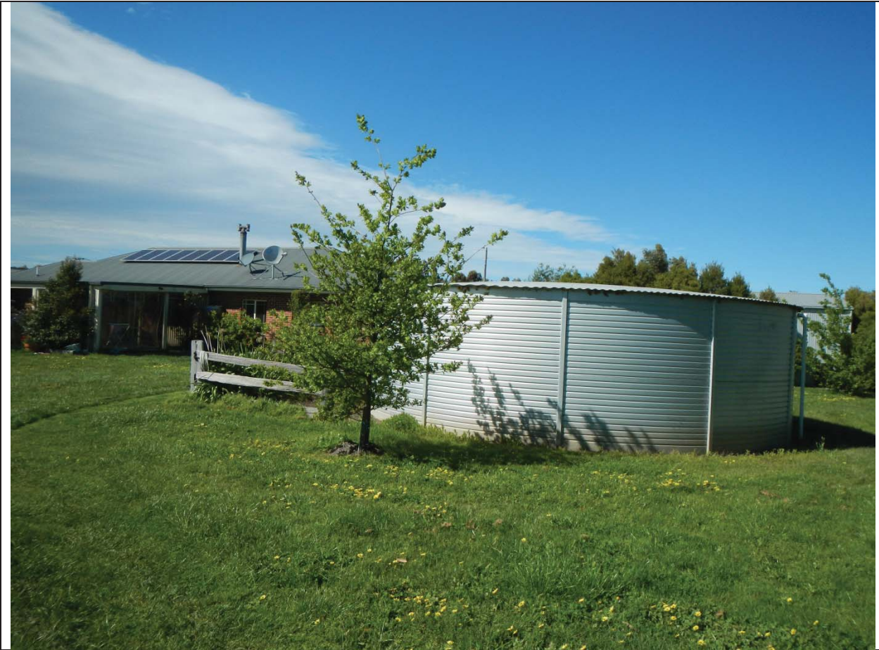
PLATE 9 Rain Water Storage Tanks (South tank) (Source of WT01, WT02, WT03)
