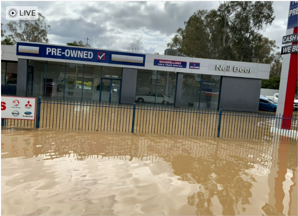
The Used Car Showroom, Seymour was inundated to a depth of 2 feet. Full renovation of this building is still not complete.
