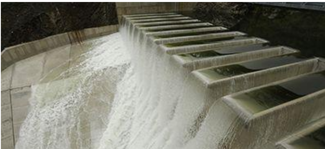
Figure 14: An example of a piano key spillway 17
