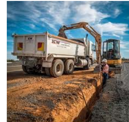
Mildura Airport Runway Upgrade
