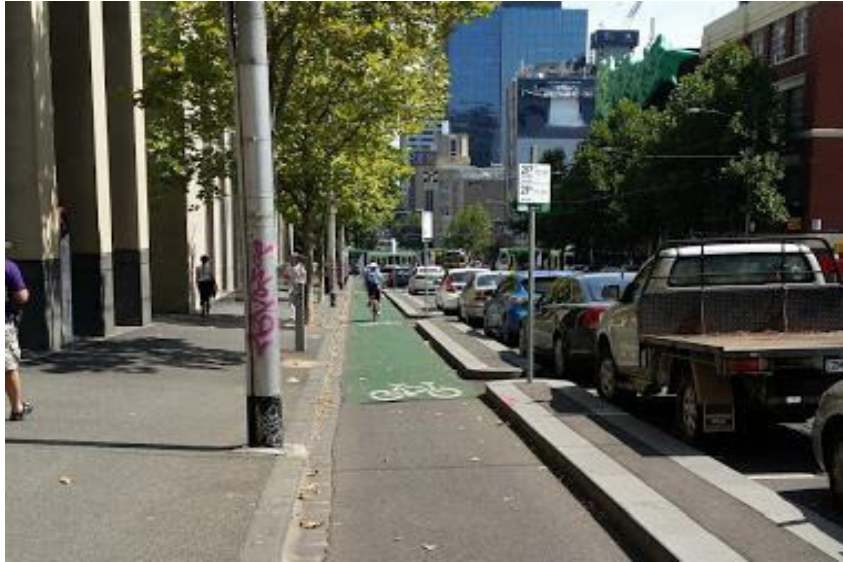
One-way protected bicycle lane on La Trobe Street, Melbourne Central Business District
