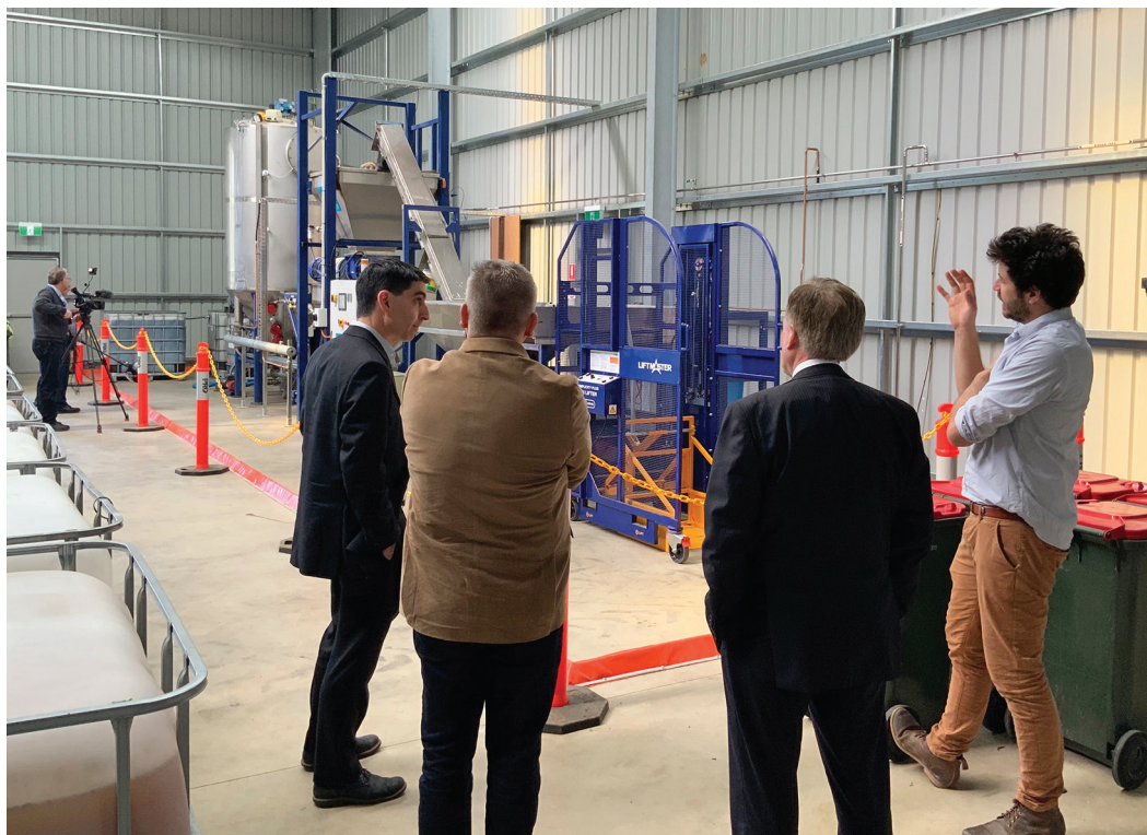
Figure 6.2 Hepburn Shire anaerobic digester
