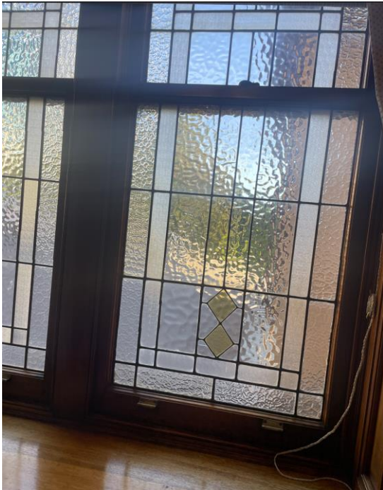
Existing heritage glazed window to be retained
