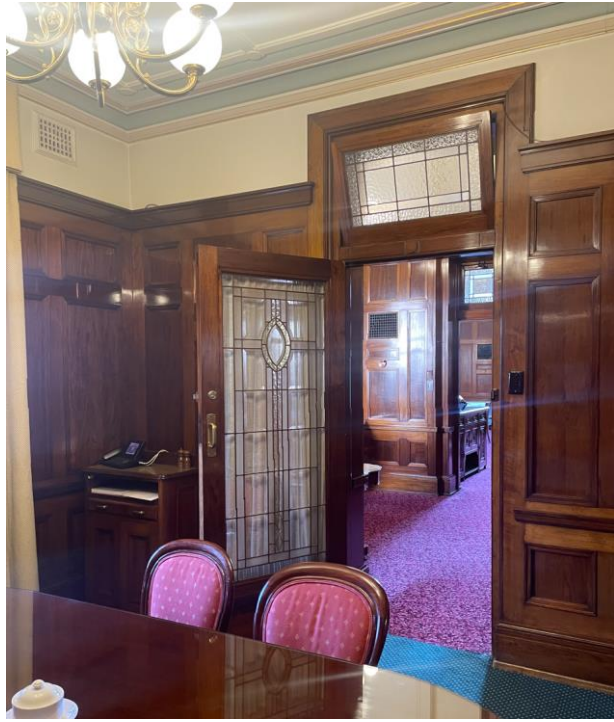
Existing heritage glazed door to be retained
