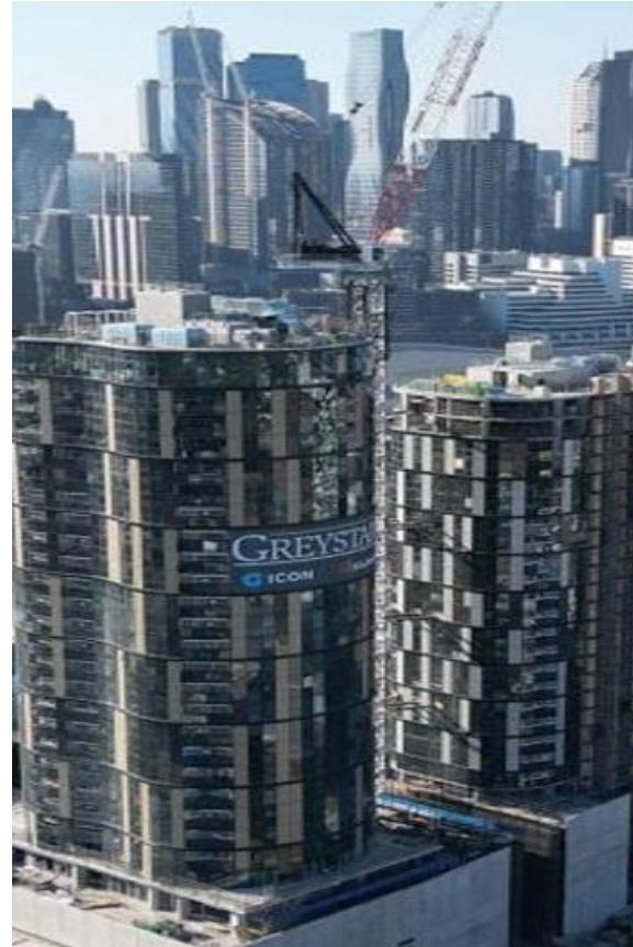
Greystar build-to-rent development (700 dwellings) under construction in Montague sub-precinct
