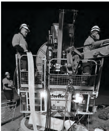
Figure 2. Renewing a crucial 750mm trunk sewer main in Bendigo
