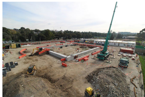
Site works at Burwood.
