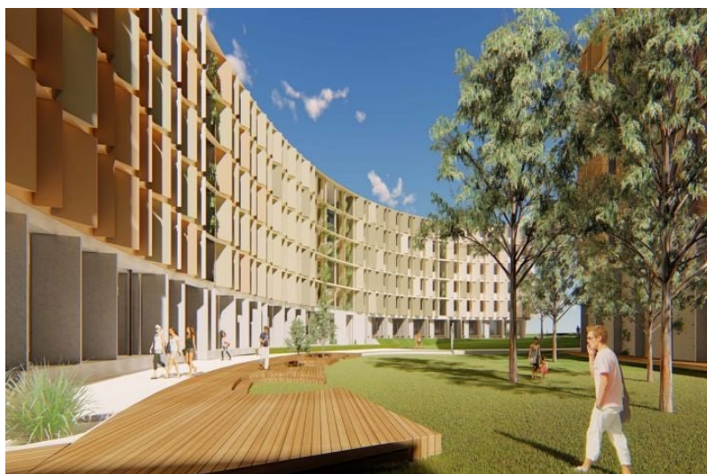
Figure 4 La Trobe University's Bundoora Student Accommodation
