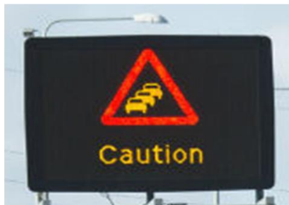
Figure 44 Typical VMS sign used to warn driver of changing conditions and increased crash risk
