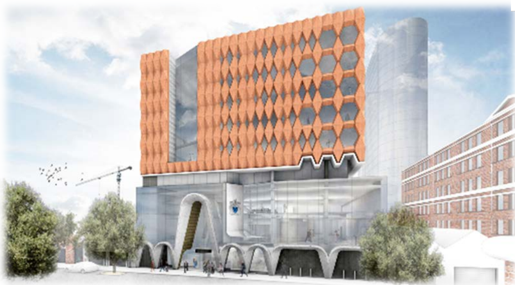
West Melbourne Custody Complex street view
