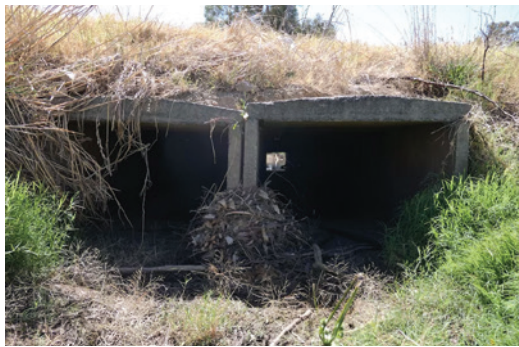
Figure 5.20 Culverts along the Murray Valley highway
