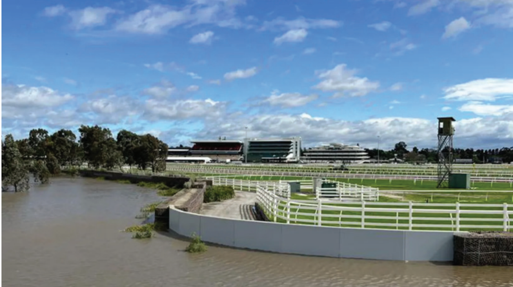
Figure 5.7 Flemington Racecourse flood wall during the October 2022 floods
