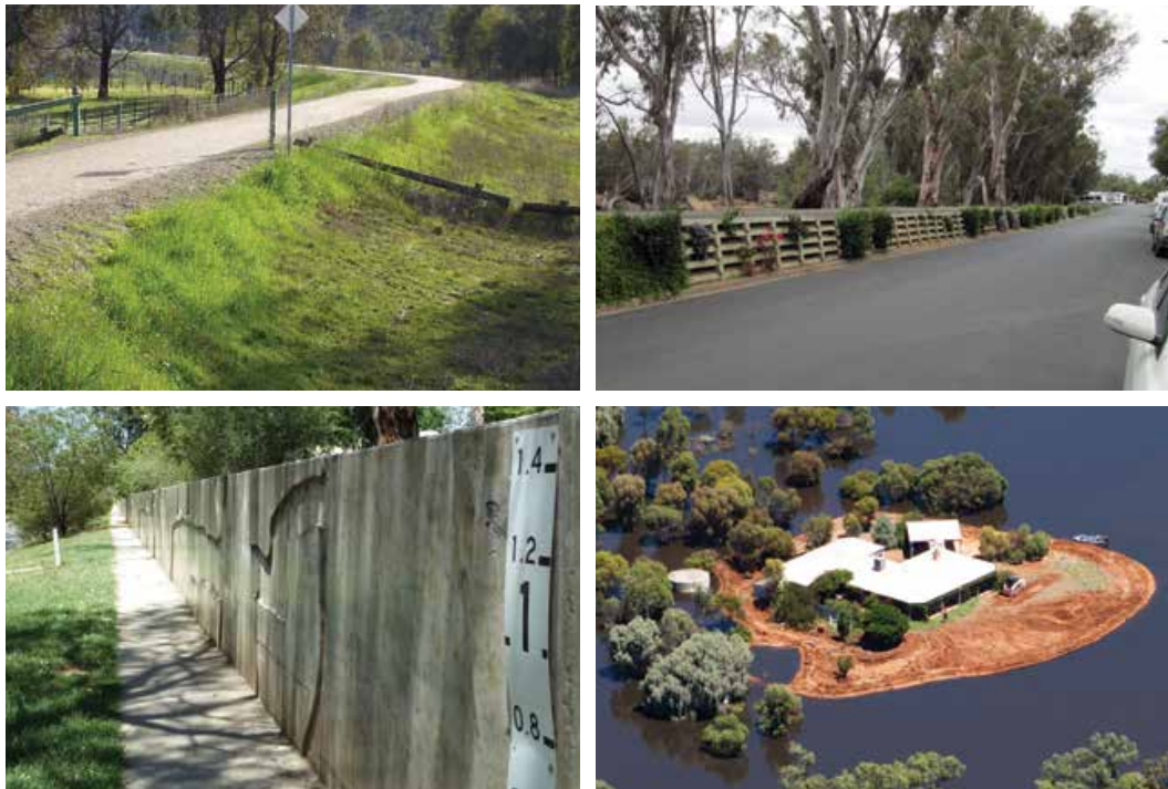
Figure 5.2 Examples of permanent levee systems
