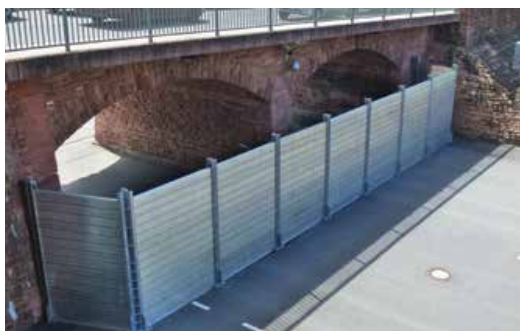
Figure 5.3 Example of a temporary levee
