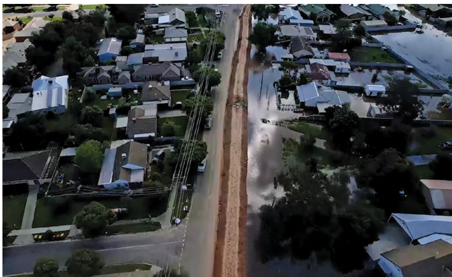
Figure 2.16 Partial aerial view of the levee and flood damage in Echuca from October 2022 flood event
