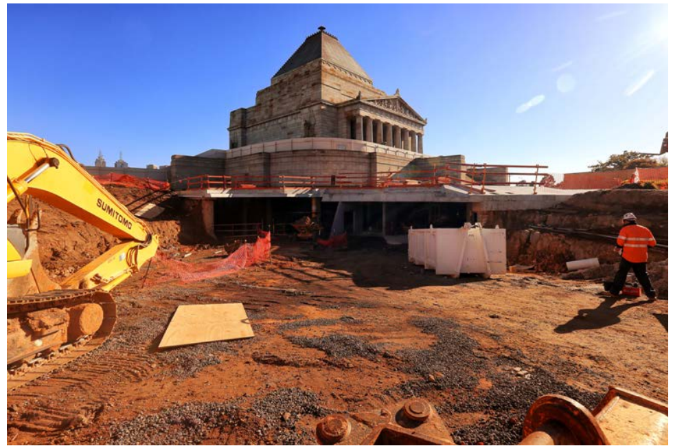
Excavation work underway for the Galleries of Remembrance
