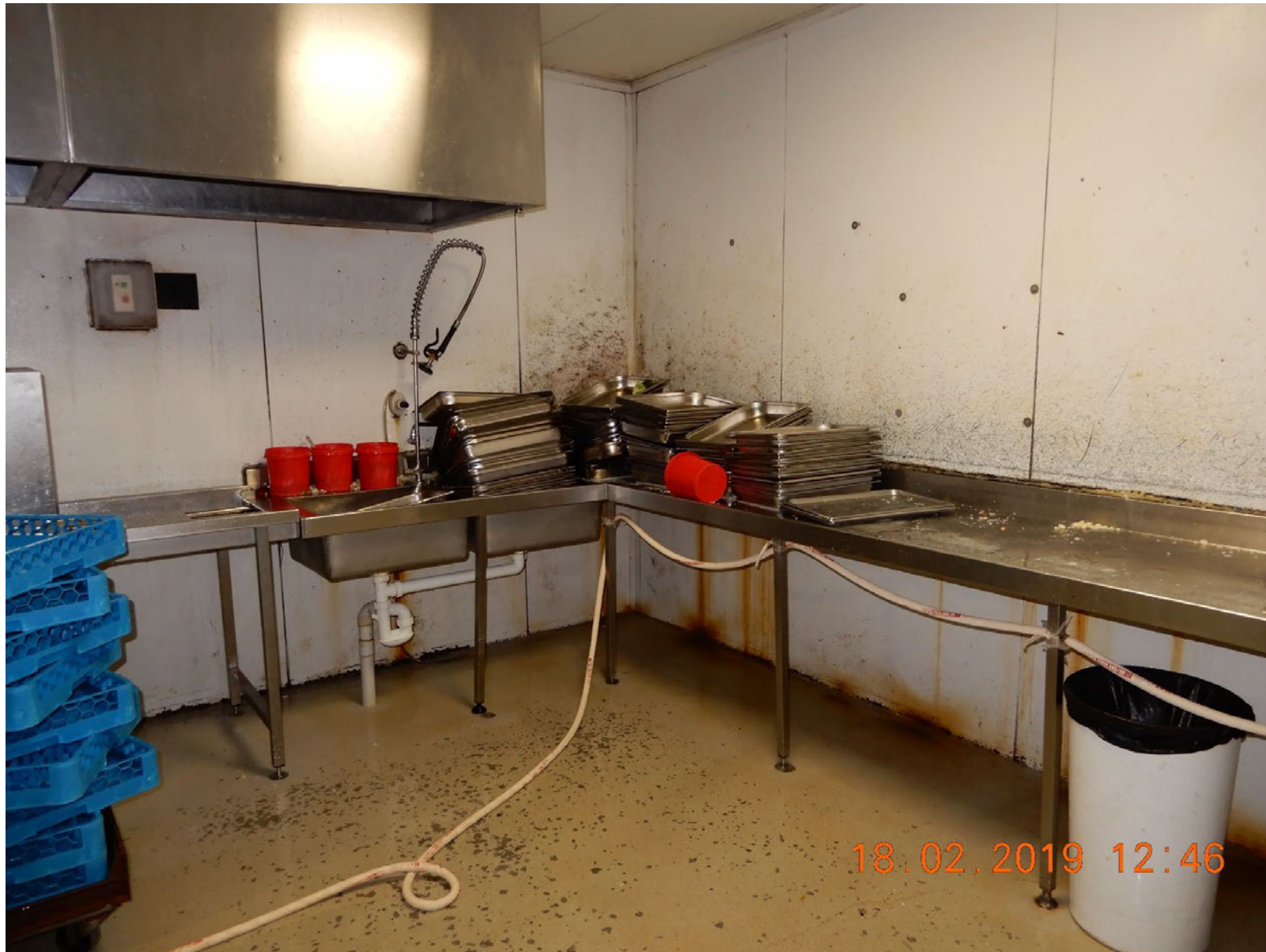
EG36: Photograph of bench and double bowl sink within Scullery Area.
