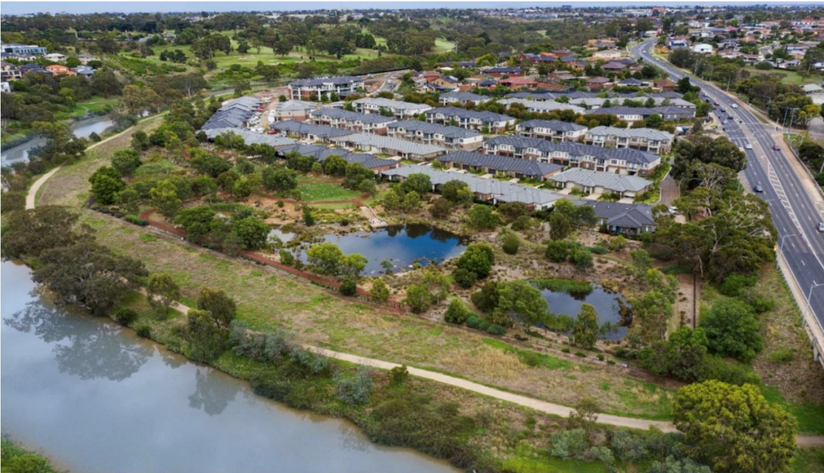
Photo of Rivervue Retirement Village, showing the constructed retarding basins in the area of the site close to the river corridor land. Canning Street is seen at the right of photo.
