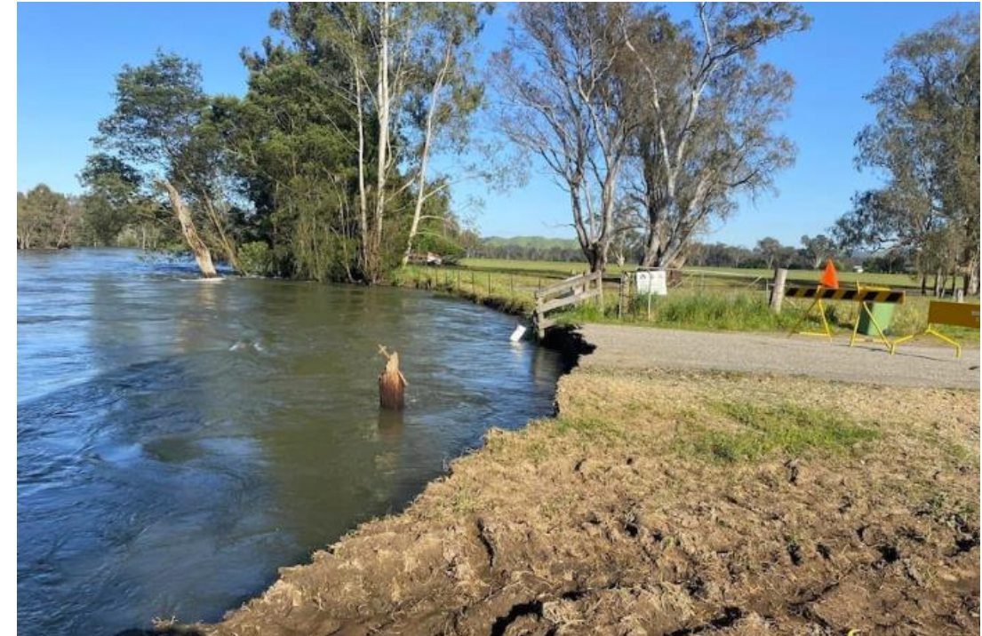
Figure 4.1: The Acheron Breakaway Bridge, which remains closed following the flood.
