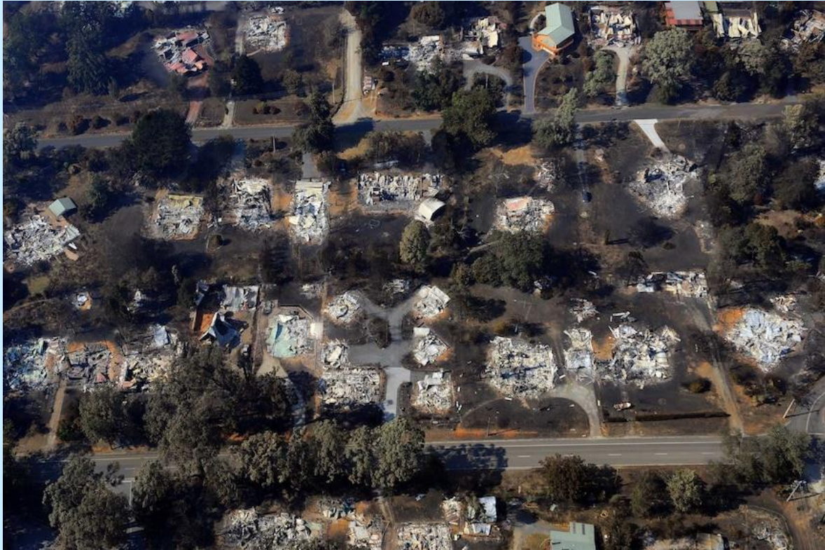
Figure 4.5: Destroyed properties in Marysville, Murrindindi Shire, following the 2009 Black Saturday bushfires.
