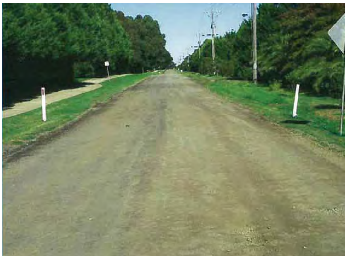
Image 1: Market Lane, Narre Warren South before the road works
